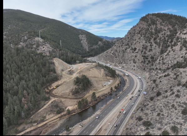
Photo of Saddle Cut construction (3/28/25)
