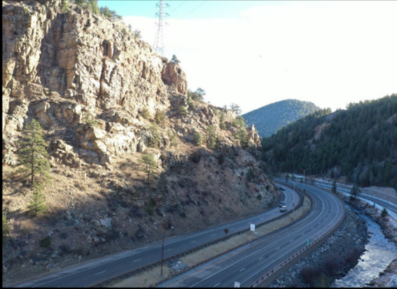
Existing Condition of I-70
