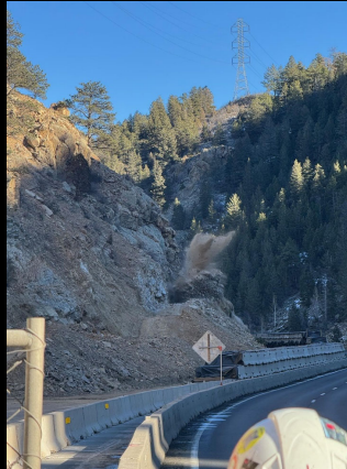
West Section rock blast
