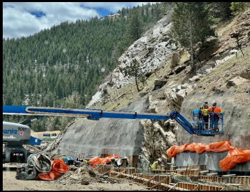
East Section soil nail walls
