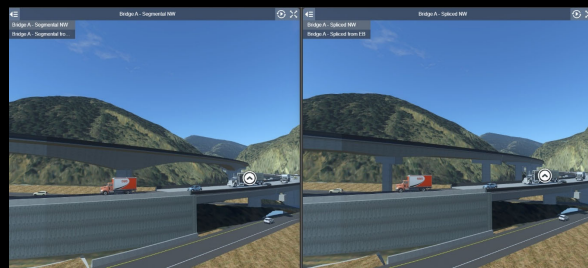
LumenRT 360 of Segmental vs. Splice Girder Bridge
