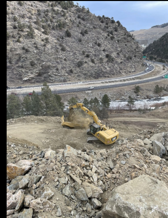
Central Section excavation
