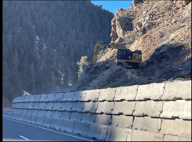
Photo of Rock Scaling (12/20/24)
