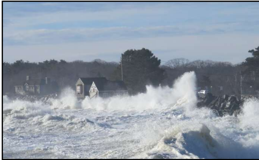
Coastal Revetment Reconstruction
