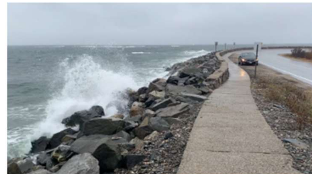
Route 1A in Rye, NH (Photo Credit: GZA)
