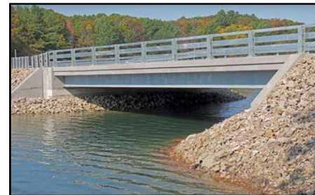
Bridge Replacement and Approach Road
