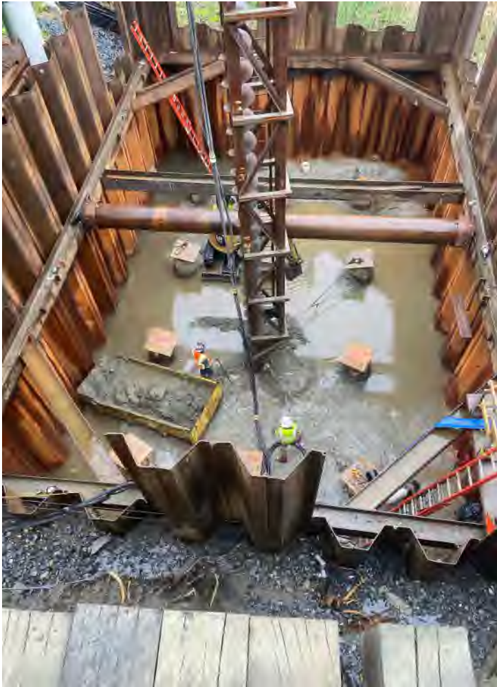
Multiple Cleanout Methods: Auger w/ Flighting, Air Lift, Soilmec Auger
