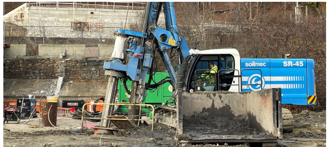
Multiple Cleanout Methods: Auger w/ Flighting, Air Lift, Soilmec Auger
