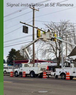
Signal installation at SE Ramona
