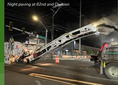
Night paving at 82nd and Division
